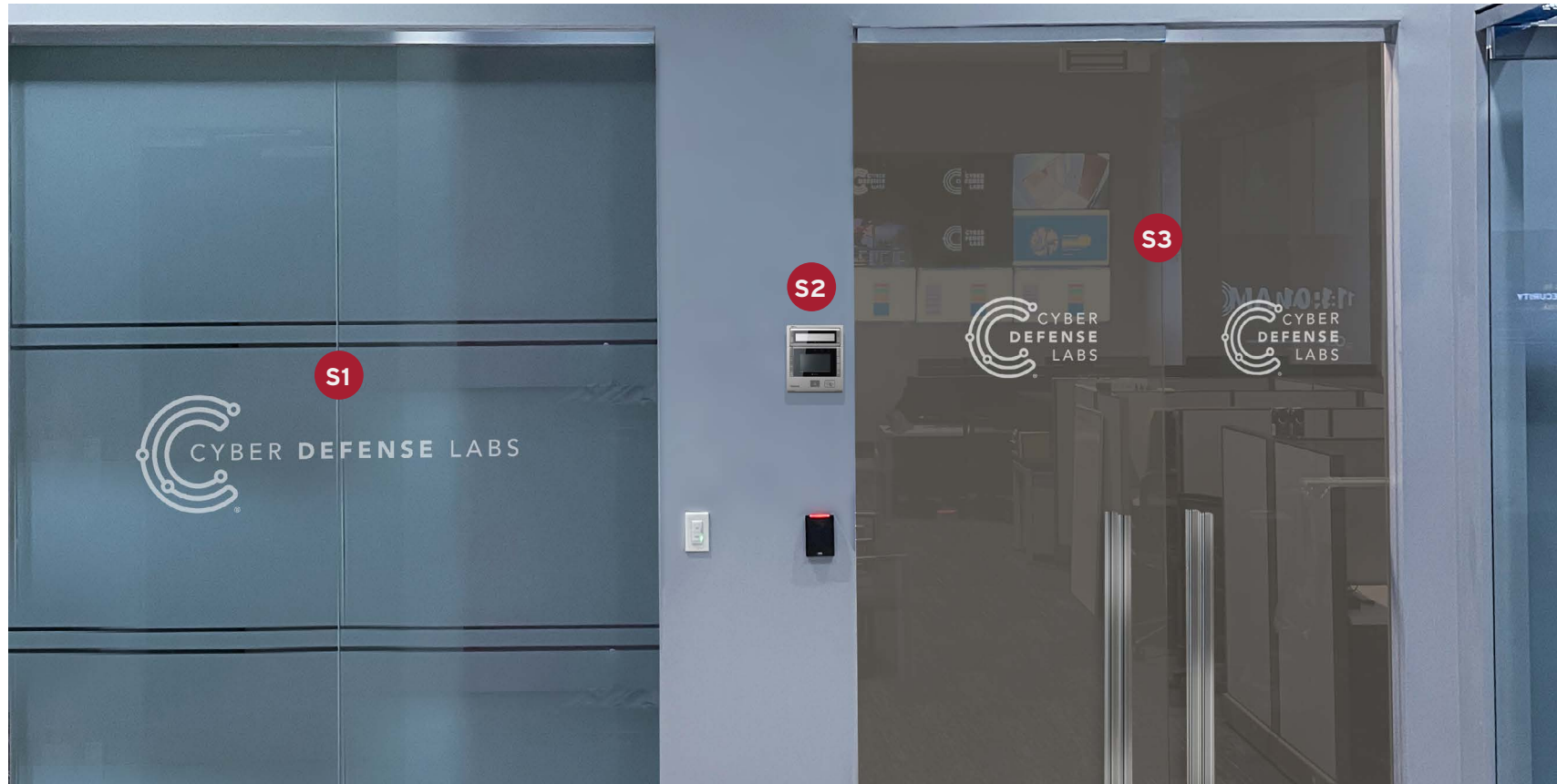
SOC office windows and doors. Retina and face scanner.
